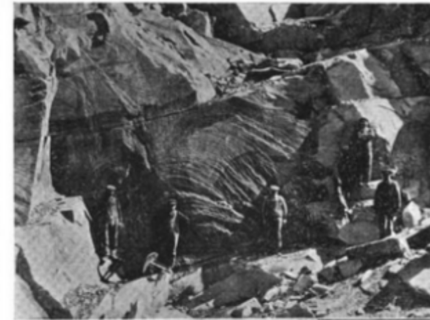
This is a view of Smalley's Pink and Imperial Red Westerly Quarries where the rough stock for the Titanic Memorial was quarried.
