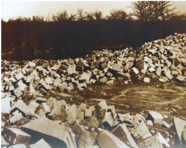
Rip rap, granite waste used to build sea wall after 1938 hurricane
