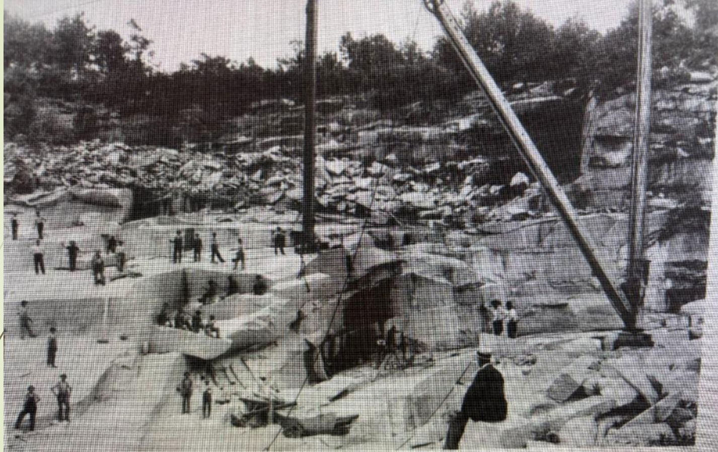
Figure 7. New England Granite Company Quarry No. 1, published in Merrimack County Art Work, 1893. At left of center, two rows of quarriers coordinate their drilling, apparently oblivious to a large block of granite about to be lifted past them. This quarry was engaged at the time in supplying granite for the Library of Congress, the largest building project anywhere to that date. In 1896 the company employed 85 quarrymen, 154 granite cutters, 40 laborers, 2 machine men, and 12 tool sharpeners. Courtesy of the Concord Public Library. F4197.
