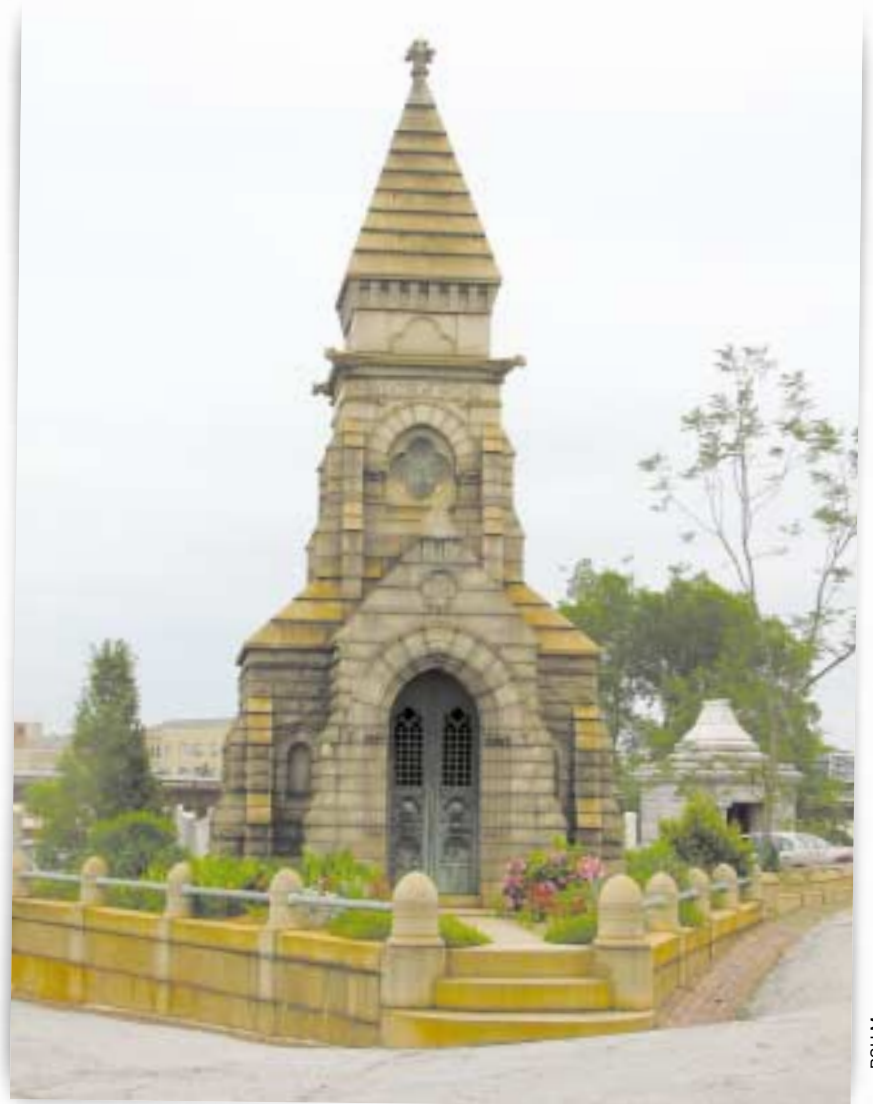
The Richards mausoleum, gothic in style, is a focal point of the Oakland Cemetery in Atlanta, GA.
