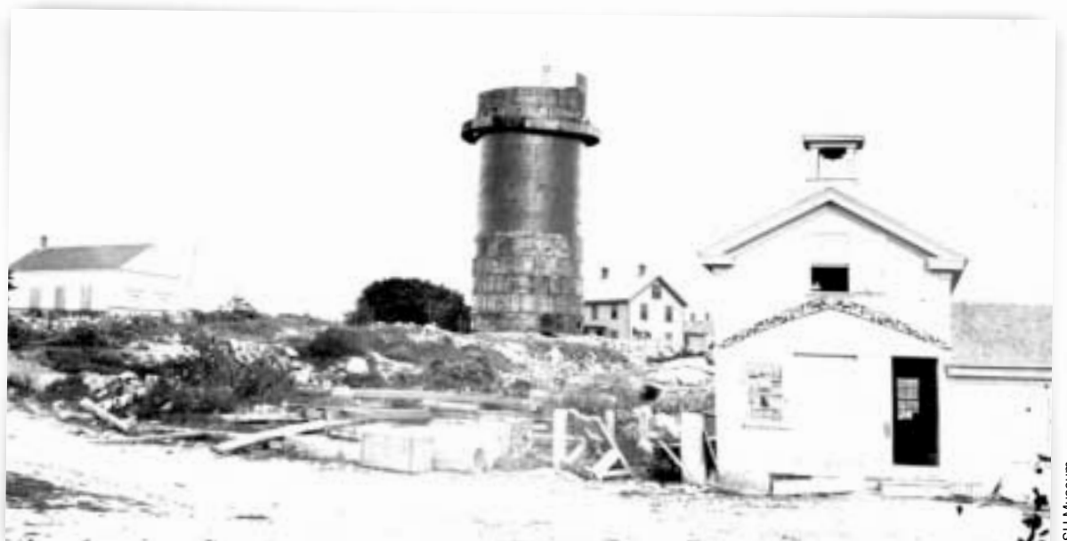
Preparing for the new Smith Granite Company Store circa 1882. Water Tower under construction, Gourley House behind water tower. Old company store in right foreground. Building materials for new store center foreground.
