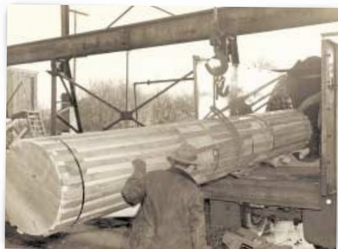
Louis Giorno at the Smith Granite Company with a large cylinder turned with the lathe and packaged for travel
