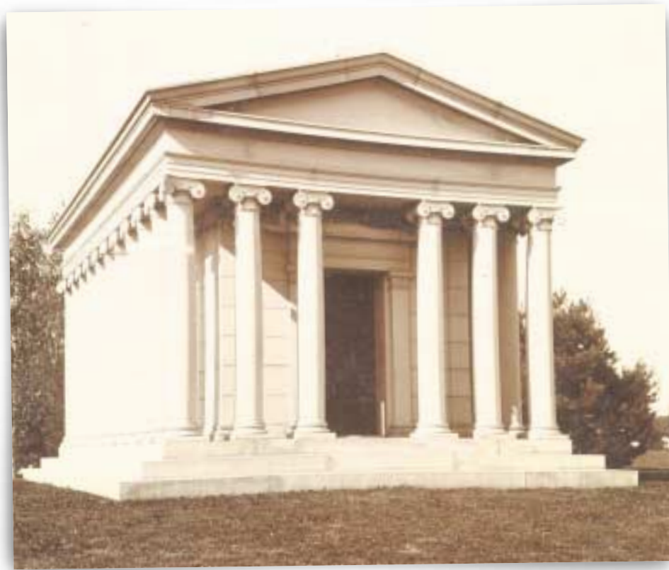
The Gould Mausoleum in Woodlawn Cemetery in the Bronx was produced by the Smith Granite Company from Westerly blue granite in 1893. It features 30 Ionic columns, each 18 inches at the base and 18 1/2 feet tall, on all four sides, 32 crypts, and two levels inside.
