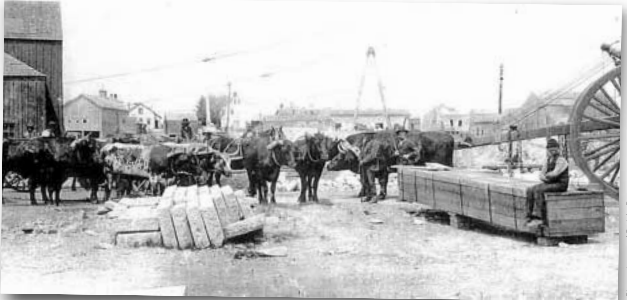
Oxen at New England Granite Works, looking north. Houses in the background are on Ledward Avenue. Notice the large high-wheel cart in the right foreground. The wheels are twelve feet in diameter.
