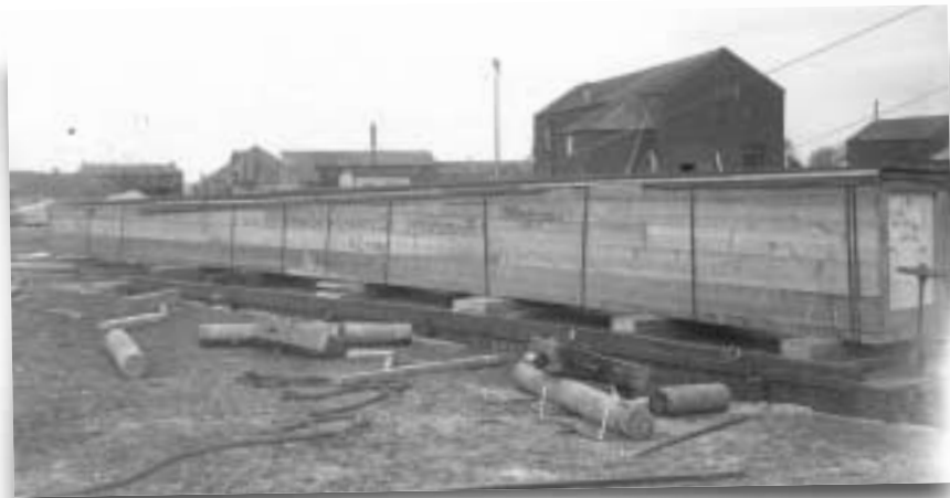
The Hall Shaft boxed and on a railroad car, ready for the railroad trip to New York City. This monument was so long, nearly 50 feet, that the end of the monument overhung the railroad car; an empty car had to be coupled to this one to accommodate the swing.
