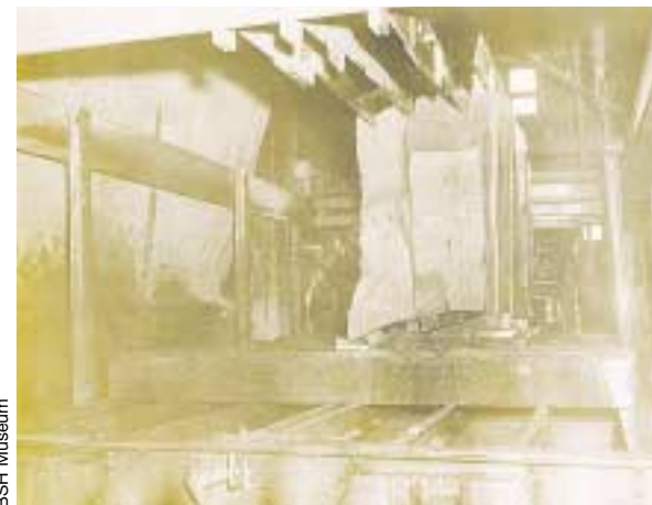
The Smith Granite Company had the first gang saw in Westerly. It was a very noisy operation that affected the hearing of the operators and, therefore, was run at night. If anyone has a better picture of the gang saw, we would love to have a copy.
