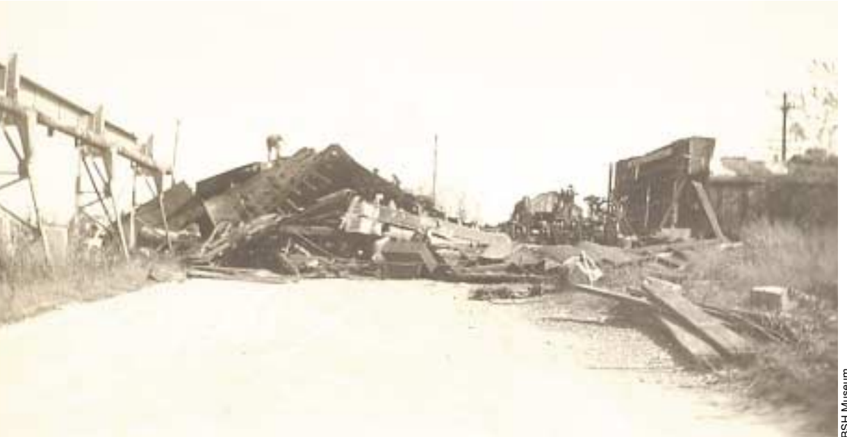
Damage to the Smith Granite Company from the September 23, 1938 hurricane. Some machines still stood after the storm. In this photo some wreckage has already been cleared and a section of one side has been braced up.
