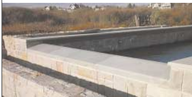
This picture shows Westerly Blue granite being used as a pool coping and infinity edge along with Westerly Pink veneer wall stone in new construction of a home in Westerly. Each stone hand worked to perfection by local mason Fred Lindsley.
